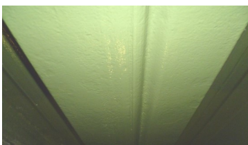
Submerged marine infrastructure
