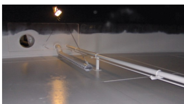
Interior crude oil storage tank
